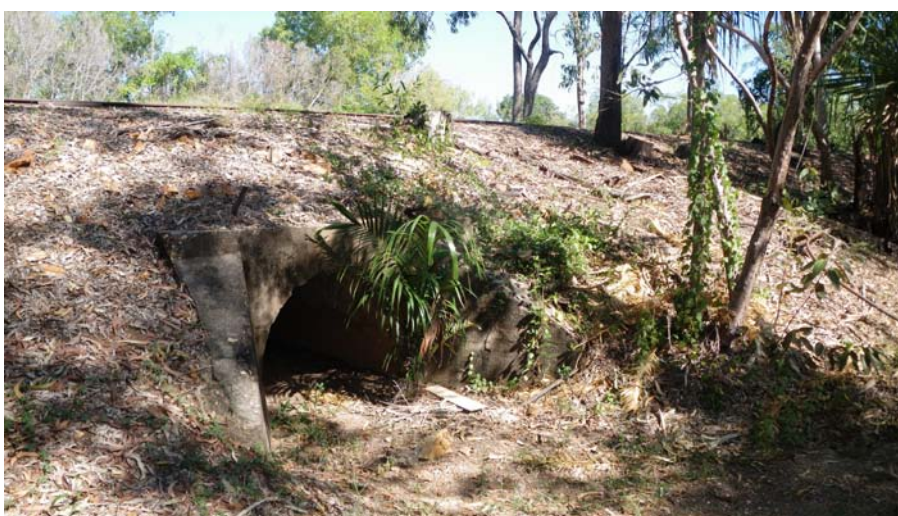
Plate 9. An original concrete drain which passes underneath the embankment.
