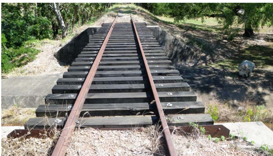
Plate 5. Top of the railway bridge showing the recently installed timber sleepers.
