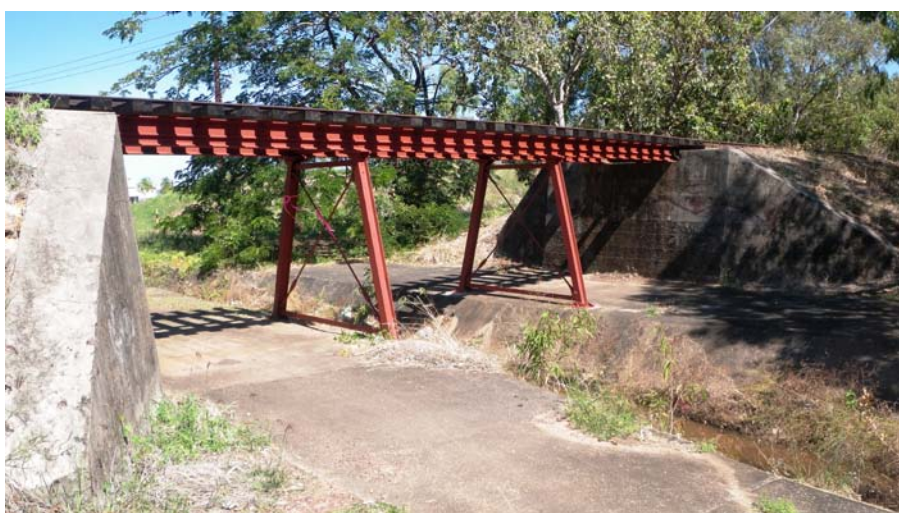
Plate 6. The recently repainted railway bridge made from Dorman and Long steel.
