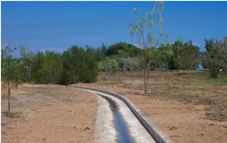
Photo H Concrete invert open drain. Surrounding areas graded to flow into drain. Dry season flows directed to lake.
